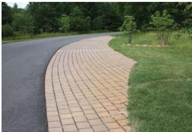
through the paving material itself or through the joints between pavers instead of running across the surface. Runoff then enters an underground stone-filled storage bed where it can be released slowly, helping to manage stormwater in a sustainable manner at its source.
