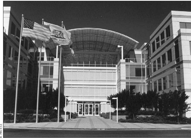
By allowing the transfer of rights from three separate sending sites, Cupertino, California was able to approve an office park for Apple Computer on this receiving site without overburdening the City's transportation system.
