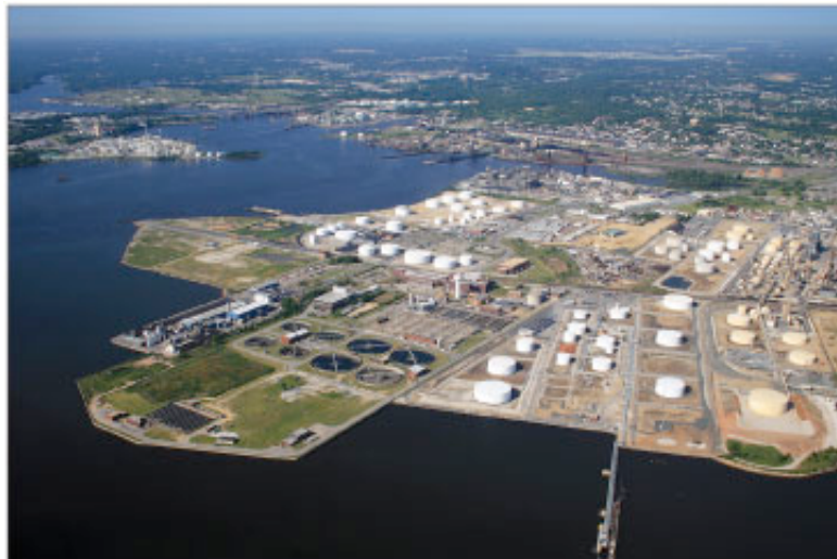
View of the Patapsco River, Baltimore, including oil tank farms and the Patapsco Wastewater Treatment Plant. Curtis Creek is in the background. Photograph by Jane Thomas, IAN Image Library ( www.ian.umces.edu/imagelibrary/ ).
